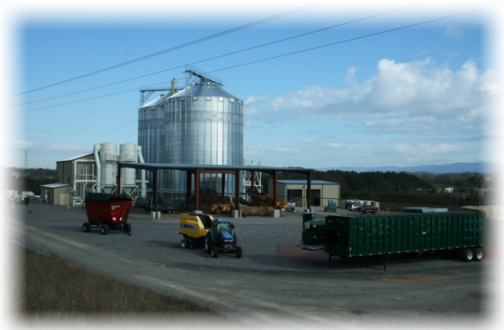
Genera's Biomass Innovation Park in Vonore
